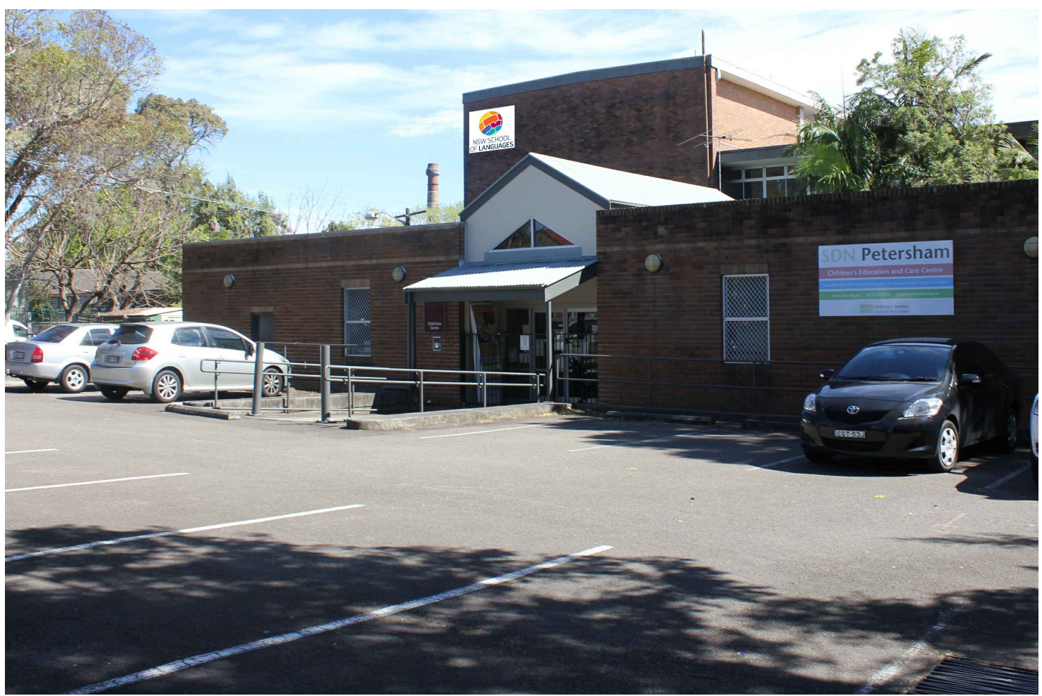
4 SIGNAGE - BLOCK A - SOUTH FACADE -
